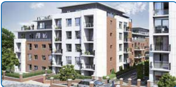
An artists impression of the completed Putney Square site, courtesy of Barratts
