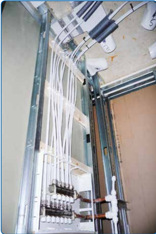
The completed installation, post pressure testing and pre-plasterboarding.
