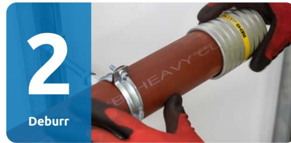
Deburr the tube using an appropriate de-burring tool or file, ensure that the external and internal of the tube end is completely free from burrs, flaps of cut material, or sharp edges.
