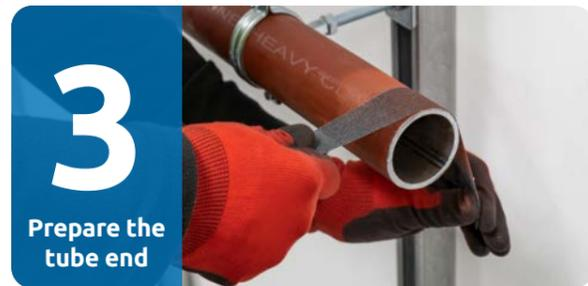
Prepare the tube end if the area of the pipe to be inserted into the fitting exhibits a poor finish including corrosion, damage, pitting, flaking, scrapes or stampings. The circumference of the tube must be thoroughly prepared using an appropriate fine abrasive pad, wire brush or flap disc.
