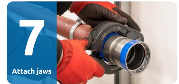
Select the appropriately sized pressing tool which can be either a jaw mounted on the press gun, or a loose collar or ring which will need an adaptor mounted on the gun. Open the jaw or collar and locate the pressing profile over the raised pressing surface of the fitting, which houses the O-ring and Anchor Ring.
