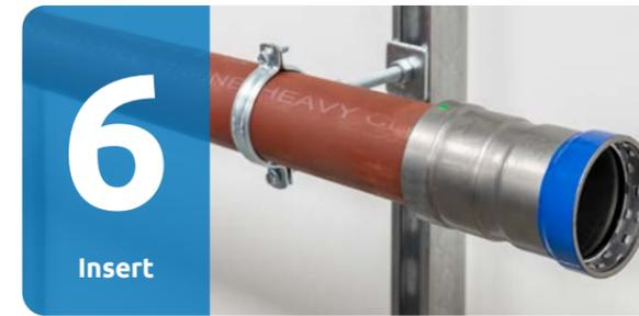
Insert the prepared tube end into the fitting and apply even pressure to fully insert the tube to the correct depth, ensuring that the fitting is kept aligned parallel with the axis of the tube throughout the operation.
