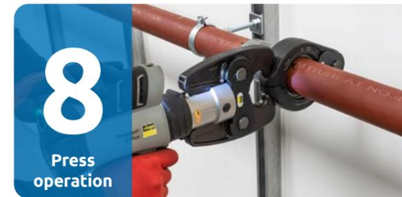
Check that the press jaw is set correctly around the pressing surface. Activate the press gun by holding the trigger or button constantly until the press cycle is completed, after which the piston will automatically retract. Once this is retracted the jaw can be opened and removed.
