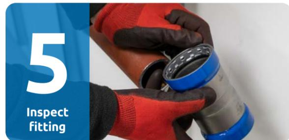
Visually double check the fitting before inserting the tube. Check that the O-Rings are free of damage, dust, dirt or debris.
